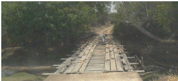
Fixing the bridge over the Ntemwa
