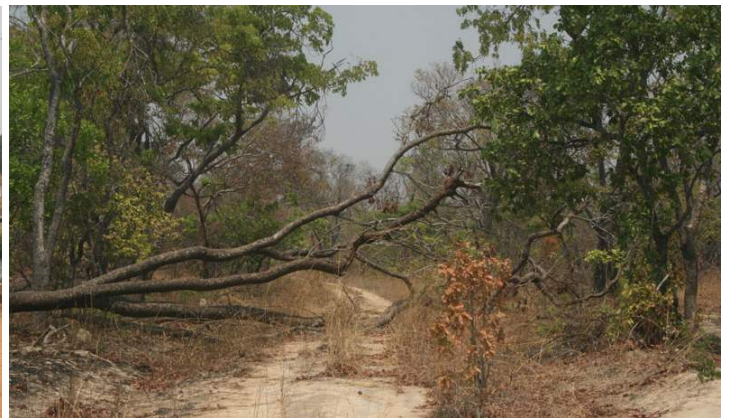
Road block on the Kabanga Road
